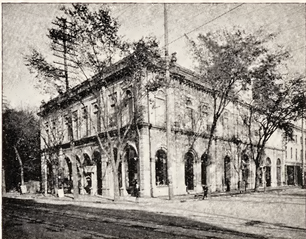
THE ART ASSOCIATION BUILDING, MONTREAL.
